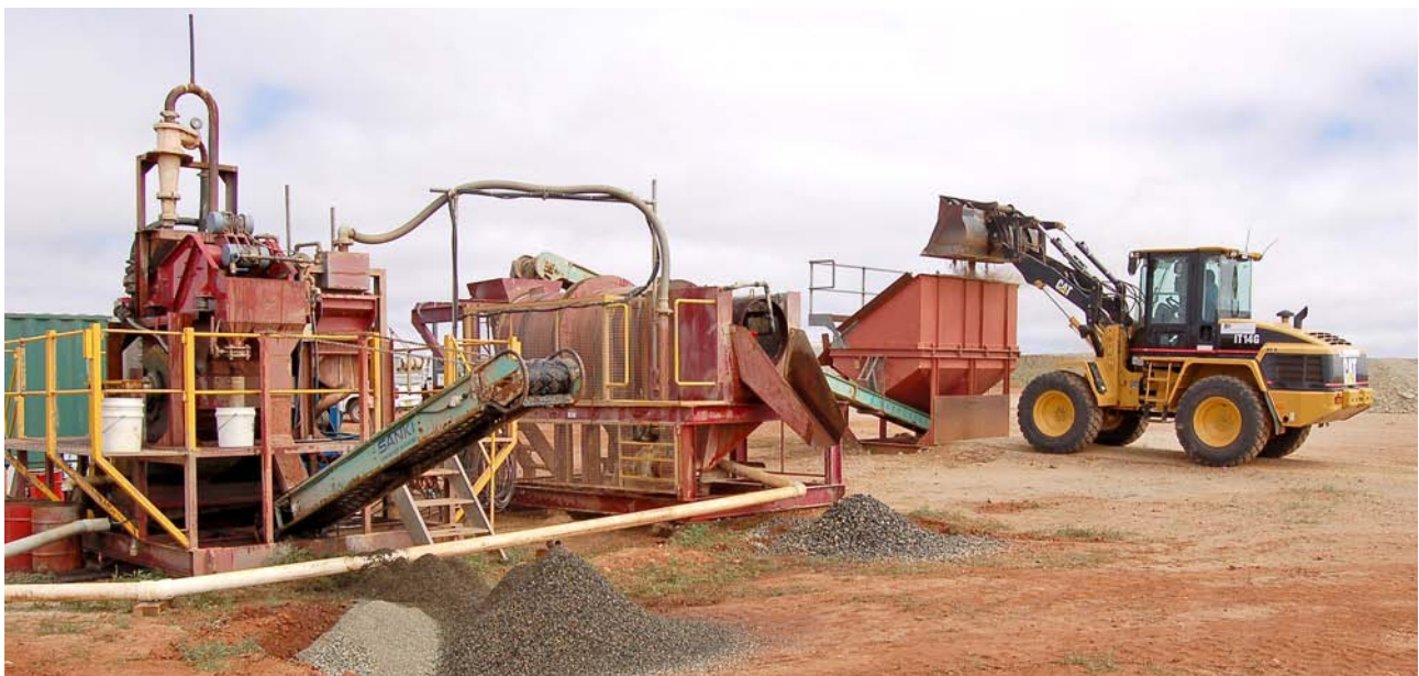
Figure 1 Bulk sampling Plant 21 during recent operations near Terowie. From right, kimberlite is loaded into the hopper via a front-end loader – then in the central trommel the kimberlite is washed and disaggregated. It then passes to the DMS (Dense Media Separation) section on the left and the heavy mineral concentrate is collected in white plastic buckets. The concentrate is then processed by laboratory x-ray sorting for diamond recovery.
